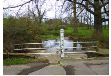
*The ford at Whitehall where the pipes beneath the road are too small.*
